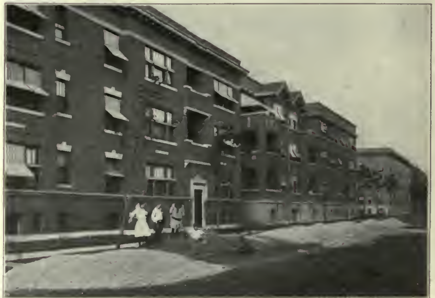
FIG. 50. STREET CONSTRUCTION, A SOURCE OF DUST. Material is frequently piled in the street where passing vehicles grind it to powder, which is quickly taken up and borne away by the wind.
